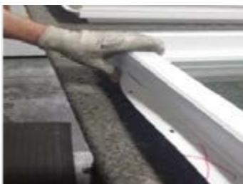
B. Remove marked nail fin(s) by scoring with a utility knife. Bend the fin down then up to remove the fin from the frame.
