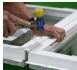
**A.** With the window interior side up, apply silicone to the first frame without the nail fin. Next, place the PVC reinforcement with silicone applied to the opposite side against window frame centered along the length.
