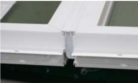
\*If there is an intersecting mull, fill intersection with silicone before applying cover
