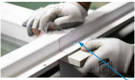
»-Then fill the rest of the cavity the same way all the way down to the bottom side of the PVC reinforcement.
