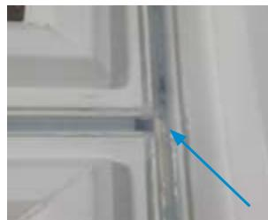
»-\*If there is an intersecting mull, first fill cavity full of silicone, then down each side of the mull channel. Also, fill accessory grove about 1" in each direction. Finally, tool/smooth silicone in all directions.
