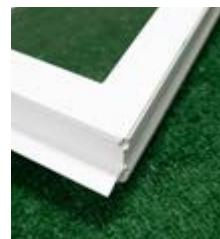
**B.** Remove marked nail fin(s) by scoring with a utility knife. Bend the fin down then up to remove the fin from the frame.
